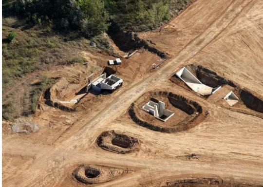
OUVRAGES DE GESTION HYDRAULIQUE TRAVERSANT ET DE POMPAGE AVANT ELEVATION DE LA DIGUE (©BRLi)
